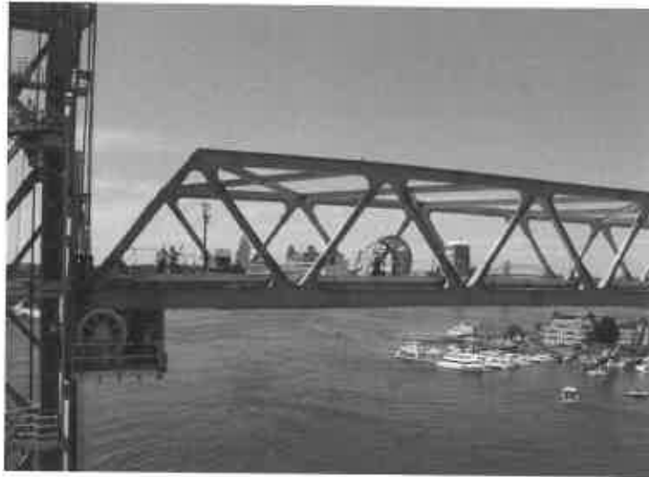
Crews at work on the lift span, MaineDOT photo.
