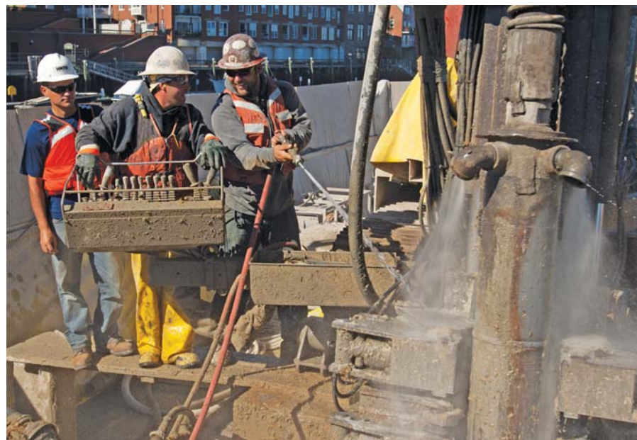
In the design of the truss, Archer-HNTB hoped to avoid one of the most problematic aspects of truss design: gusset-plate connections. The demise of the existing bridge was in no small way due to corrosion and deterioration of gusseted truss connections.
